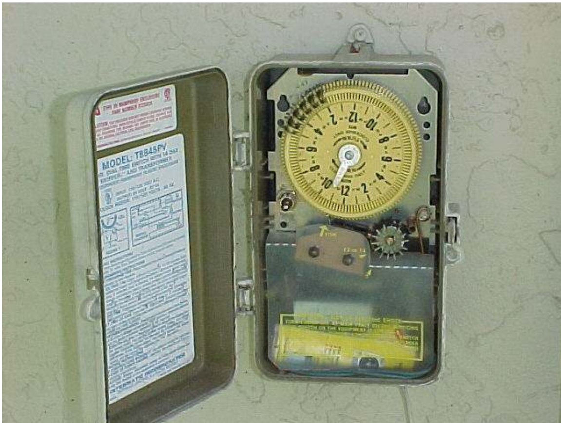
Timer for lawn sprinkler Set for 20 minutes per zone twice a week
