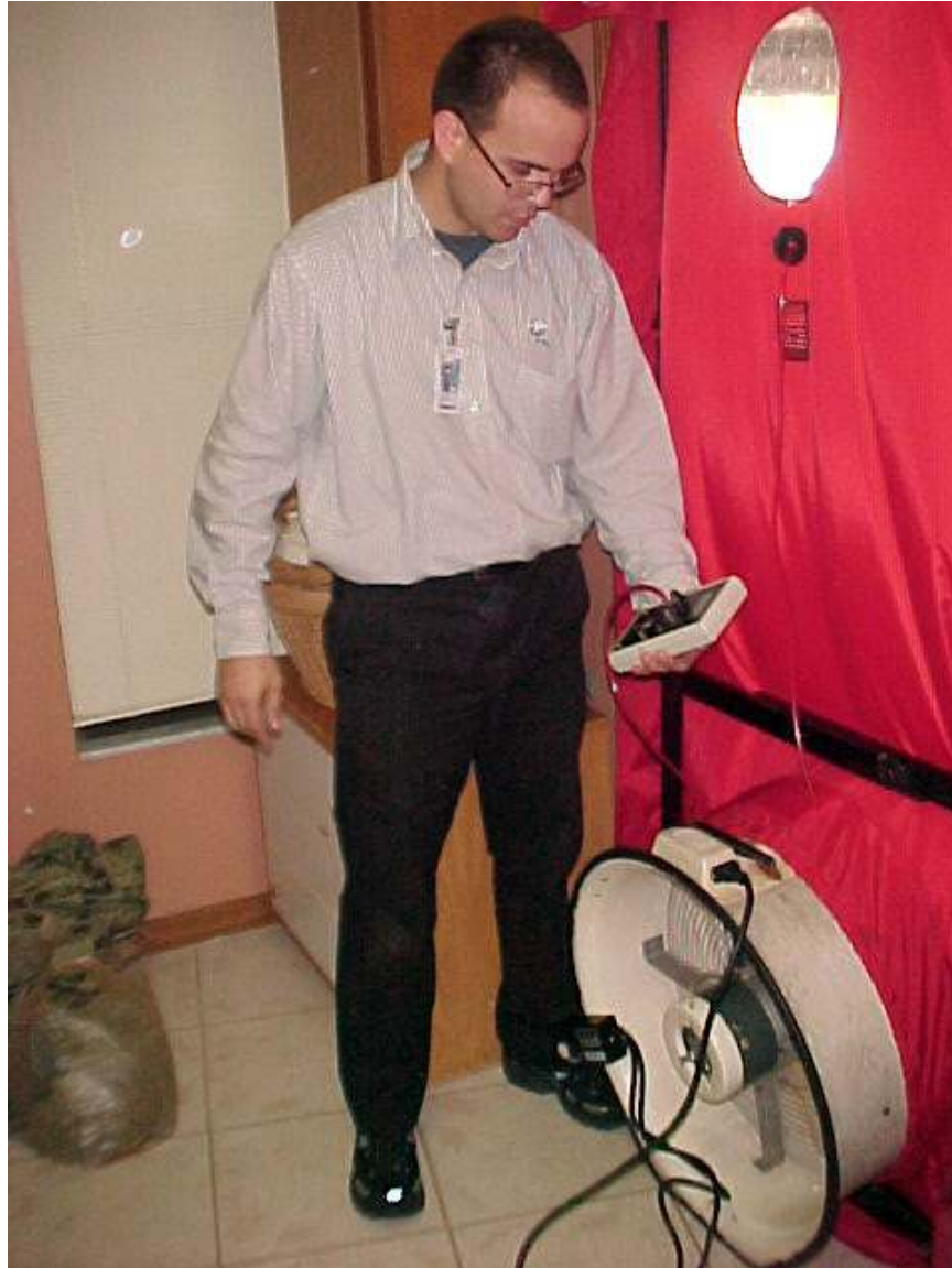
Power company inspector checks how well A/C units works by pressurizing the house.
